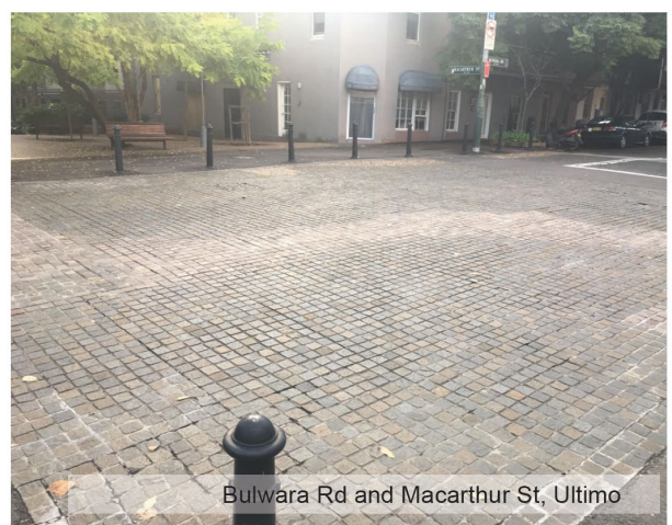
Figure 10 Special paving treatments to signalise intersections (different road material)
